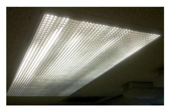
The "eggcrate" louver is composed of 1/2"Lx1/2"W squares that are 3/8" thick.
